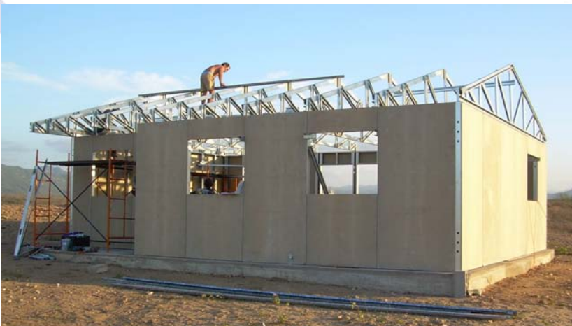
Detail roof assembly prepared for metal tile
